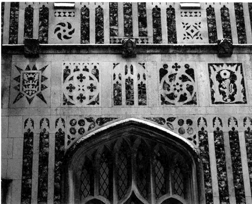
FIG. 101 – Flushwork display on the east face of the north porch at Woodbridge St Mary.
